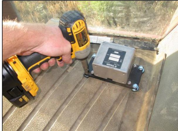
**Example: Mounting in the operator's cab**
